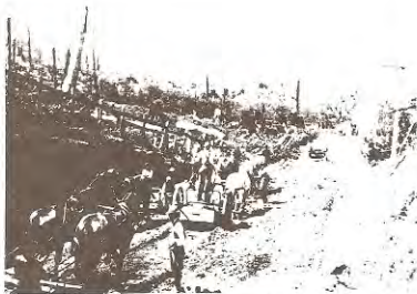
In the early days of construction
