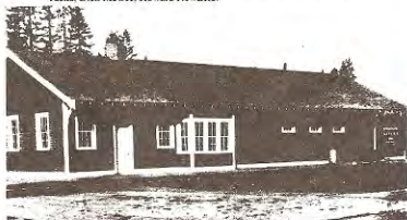
The old depot in 1920. Mr. Max Griffith preceded Mr. Osborn as depot agent. The building was later purchased by Les Mallonee, who had an electrical shop. It is now occupied by Onalaska Electric and owned by Mark Myhre.
