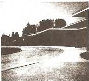
Onalaska Elementary School—built in 1958. In a campaign in 1957 for a levy for a new elementary school, the final result was a mere two votes over the required 60 percent voter approval. Mark Stodman is the present Principal, and Sharon Bower is the Assistant Principal.
